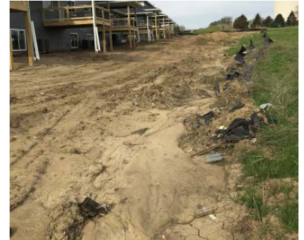
Active Work Area (does not require stabilization)
